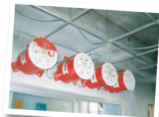
Discharged Pyrogen Generator in front of failed A/C unit
