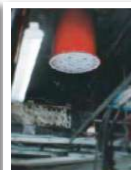
Discharged Pyrogen Generator in front of failed A/C unit
